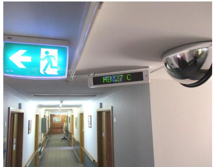
The annunciator panel is also connected to the main fire panel in the event of an alarm activation. In which case the location of the emergency is visually displayed on **all annunciator panels** located throughout the facility.
