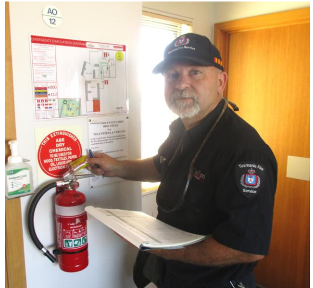
Pictured above: Tas Fire Service officer, Craig Turale inspecting one (1) of 43 fire extinguisher located throughout the facility.
