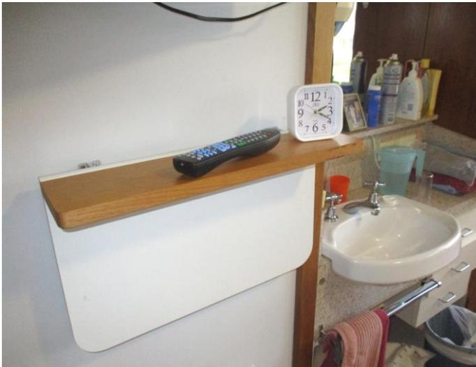
The hazard was able to be controlled by reducing the chance of hazardous contact by engineering controls. This was achieved by the shelf size being minimised to limit the overhang into the vanity space.
