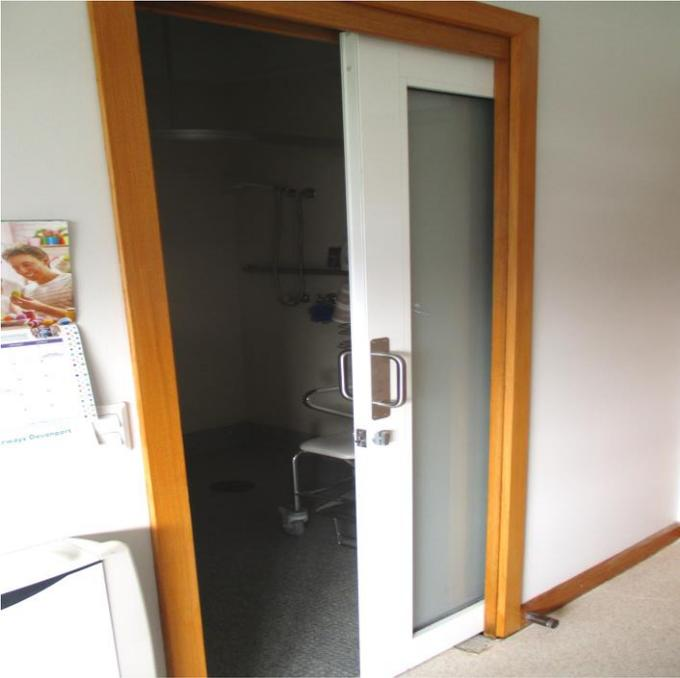
*Pictured above:* Installation of a new sliding door in Seaview. This was implemented to enable wheelchair access and assist a resident to maintain independence.
